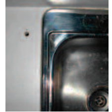
Drill quick faucet base holes
