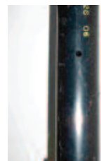
Drill hole for drain saddle assembly
