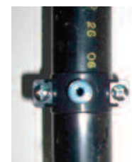
Fasten drain saddle assembly to pipe
