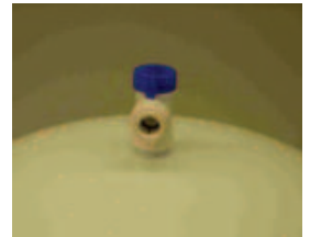
Storage tank shut off valve installed
