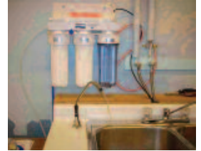
Sani Flushing the system
