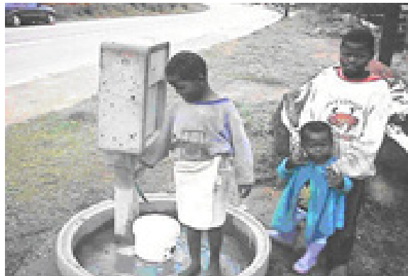
Children Filling Water from a Water Meter;
